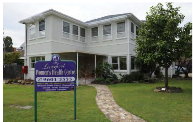
December 2010 Practical Completion
