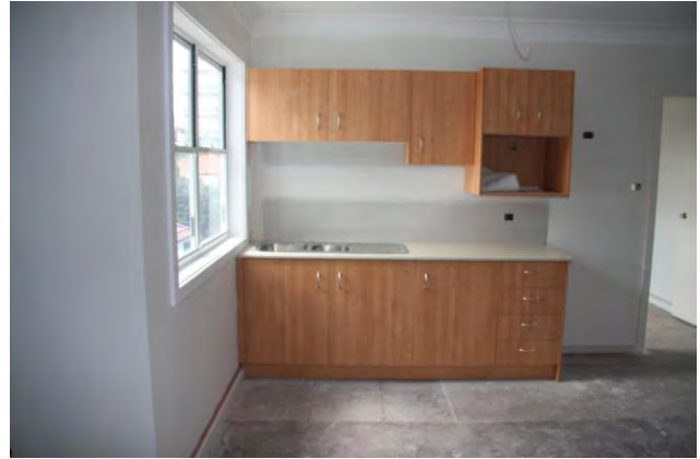
October 2010 Completion of internal fit out kitchenette
